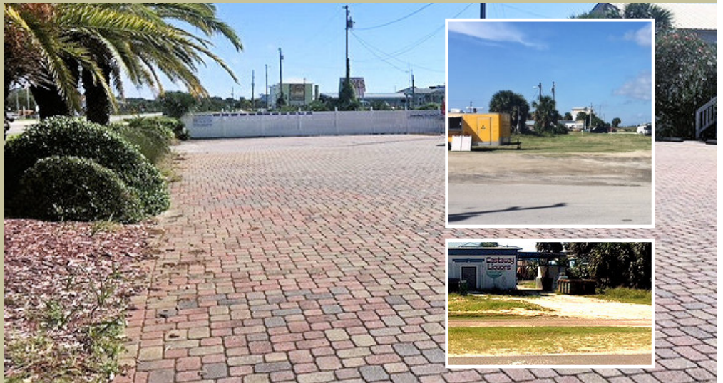
Above is an Island parking area made of durable permeable materials. Inset photos are of existing public parking area near Lighthouse Park that are unsafe, unattractive, and suffer from flooding and erosion.
