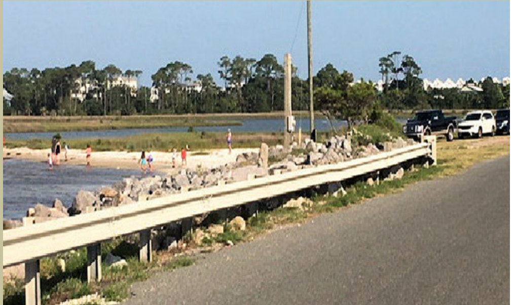
Parking and safety issues abound at the causeway entrance.
